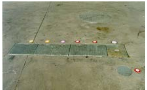
Example of coloured marking at remote fill box
