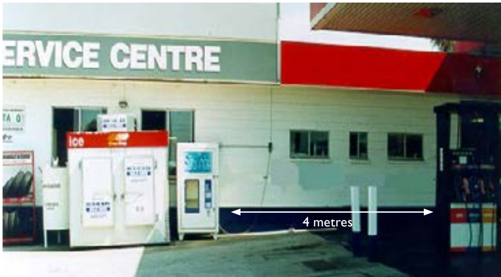
Example of minimum separation distance for dispenser from ignition source: 4 metres between fuel dispenser and freezers/ vending machines
