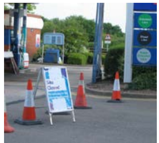
Traffic control during bulk transfer
