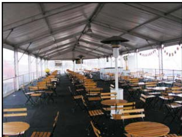
Not acceptable appliance indoors
