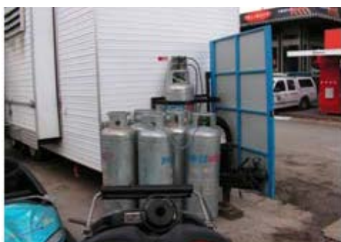
Secured to other cylinders
