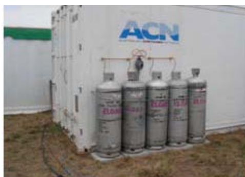
Secured and on stable base
