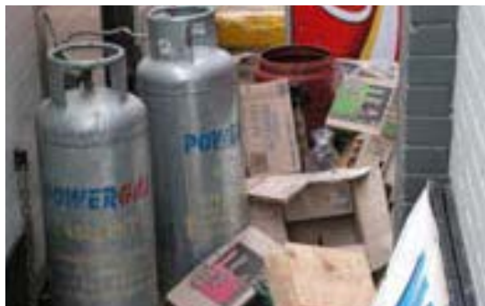
Not clear from combustibles or secure
